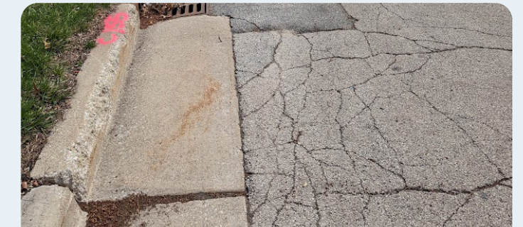
Alligator Cracking
